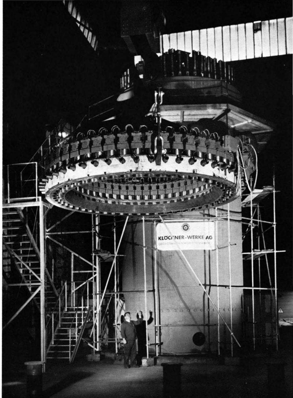
Reactor vessel for a nuclear power plant near Hamburg, supplied by the Klöckner-Werke for Siemens
